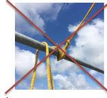
Don't attach the High-Line to any part of the structure
